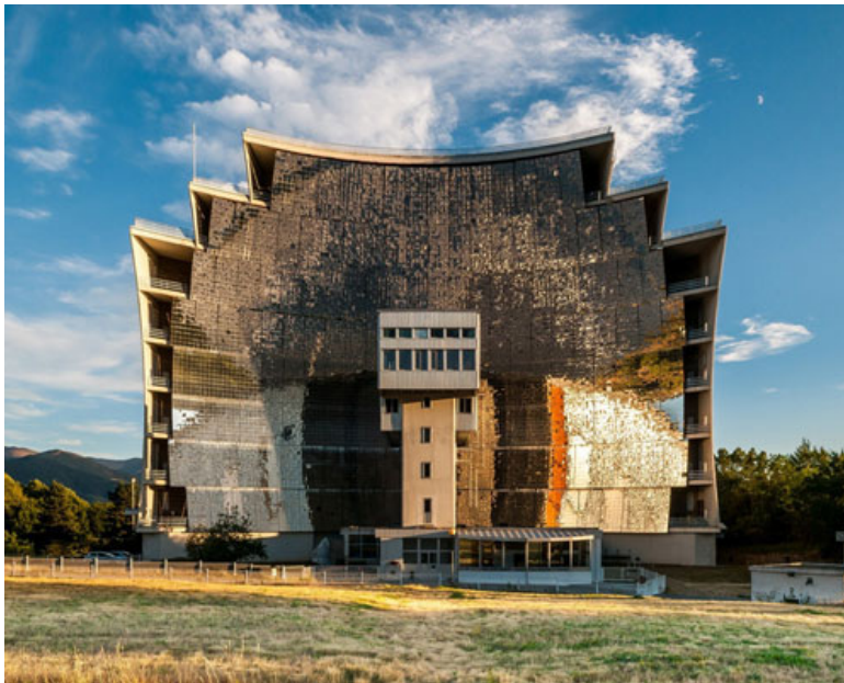
The Odeillo Solar Oven in France was opened in 1970. The site has 9,600 mirrors, focusing the sun's rays on a spot where the crucible is set to raise its temperature to 6,000 degrees Fahrenheit. Aerospace like NASA and ESA use this place to conduct high-temperature materials testing for nuclear reactors and spacecraft.
