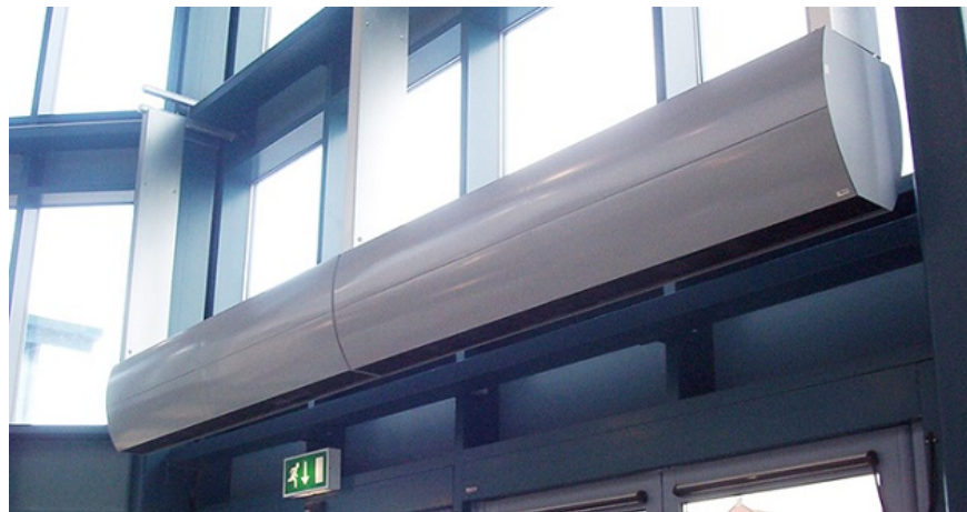
Wind-cutting fan saves electricity for room using air conditioner
