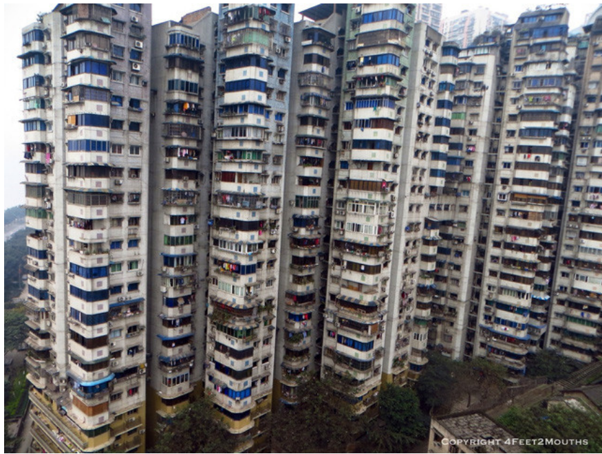
New old apartment buildings sprout up
