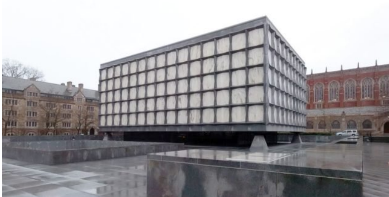
Library on rainy day, this picture depicts 4 large pillars in the corners to support the house.
