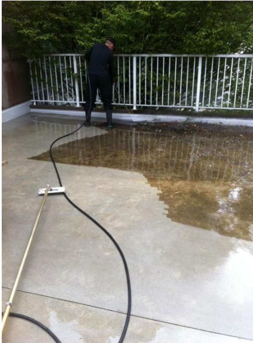
13. Add another proof of wood surface cleaning by spray pressure
