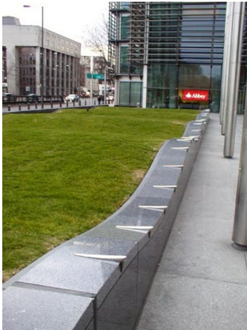
The ornament is placed on the edges of the low walls to prevent skateboarding youth.
